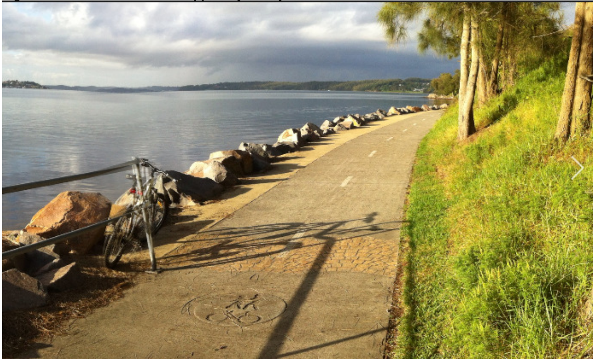
Figure 1 – Rock revetment to support cycleway construction
